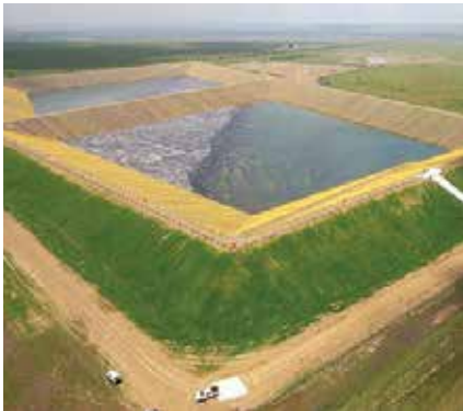
Brine Retention Pond New Denmark Anglo Coal, South Africa
