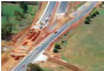
Eikenhoff R82, Provincial Road Gautrans Road construction - 800 000m 3
