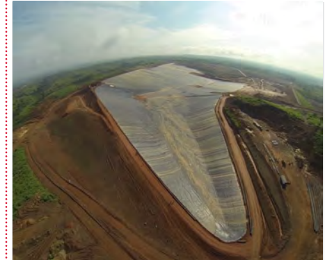
Mine Infrastructure & TSF Kibali Gold Project Randgold, DRC
