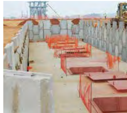
Reinforced Earth Wall with over 1 000 concrete panels to required tolerances Dorstonein Coal Total Coal, South Africa
