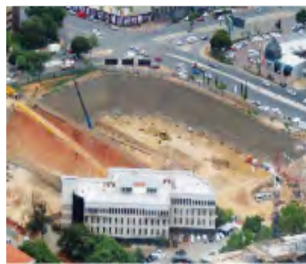
Basement Excavations Werksmans HO Sandton Investec, South Africa
