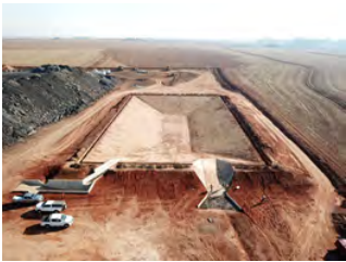
Phalandwa Colliery Canyon Coal Pollution Control Dam
