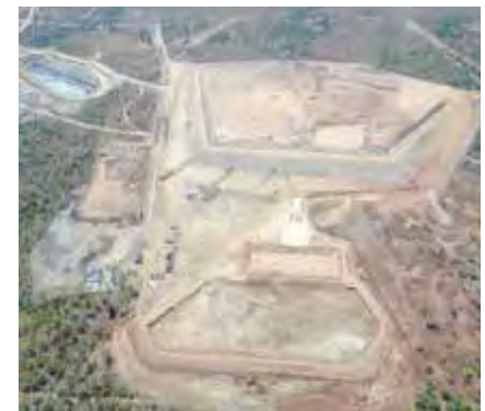
Mine Infrastructure & TSF New Luika Gold Shanta Gold, Tanzania
