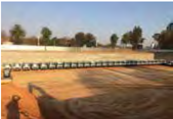
Oxford Parks Intaprop Basement Excavation 120 000m 3
