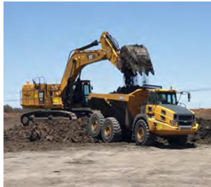
Mine Rehabilitation Kriel Coal Mine, Seriti Coal, South Africa
