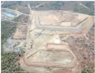
TSF, New Luika Shanta Gold Construction of Tailings Facility
